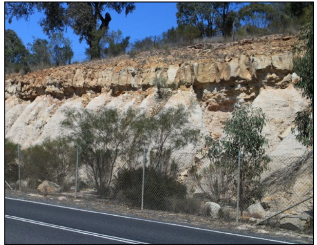
Photo 5. Weathered thin silty sandstone and siltstone beds of the Purlawaugh Formation. The thick sandstone at the top of the cutting is more representative of the Pilliga Sandstone.
