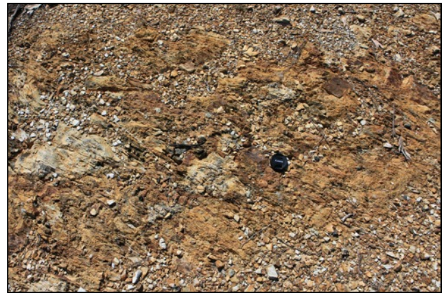
Photo 30. Cleaved weathered siltstones with iron oxide joint-fills.
